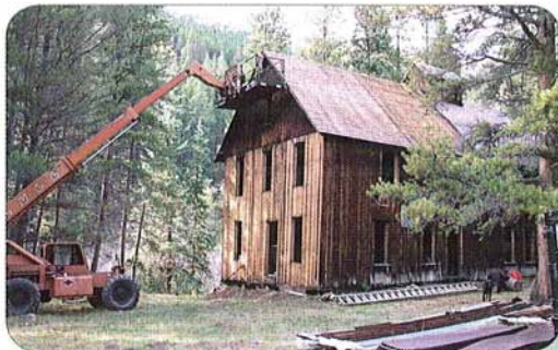
LEFT & BELOW: THE DECONSTRUCTION OF THE MINER'S BUNKHOUSE.
